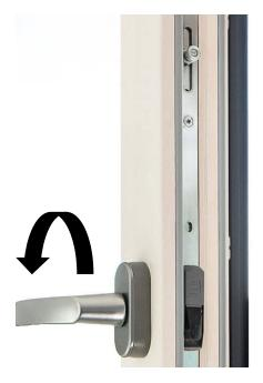
Test if the door lock assembly is functioning by pushing down on the door handle. The multi-locks should not move downward, and the deadbolt should not go back into the recess.
